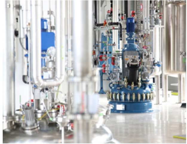
Production facility for the active pharmaceutical ingredients for innovative medicines
