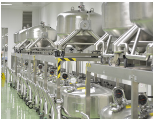
Storage containers in the Solids Ljubljana production site.
