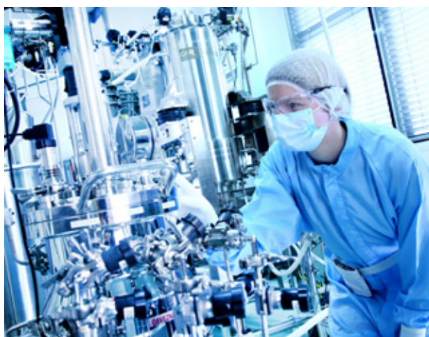
Biologics drug substances production facility in Mengeš.
